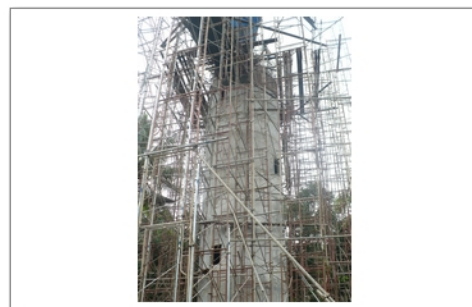
Construction of overhead water tank -23.5 million
