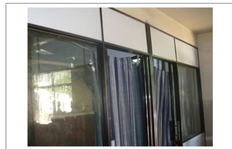
Renovation of Surgical clinic
