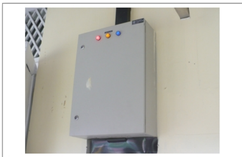
OTB Electrical repair 1 million
