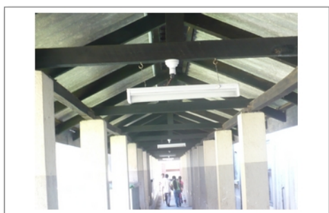
Repair of Wiring and Switch boards ( All corridors) - 1.3 million
