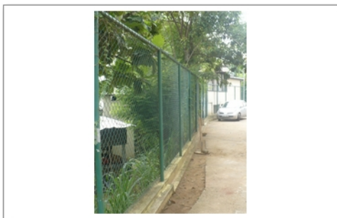
Chain link fence at the New Ward and Clinic Building 0.6 million .
