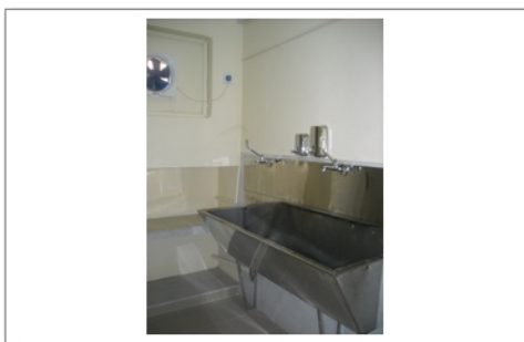
stainless steel wet basin stainless steel cloth hangers at the Surgical ICU
