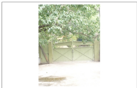
Box Iron gate and chain link fence
