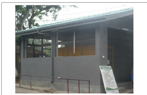
Construction of Generator room for New OPD Building - 1.35 million
