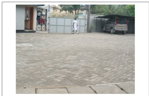
Construction of rear Gate with access and repairing of drainage System - 1.9
