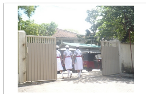
Sliding gate for main entrance at the NTS-Badulla
