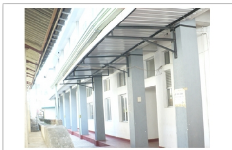
Construction of corridor ( new Drugs stores) - 1.4 million
