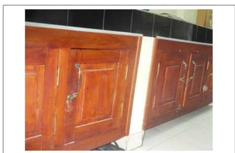
wall mounted timber shelves timber cupboard
