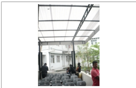
Construction of roof (balcony Mental Health Unit 1st floor) - 1.9 million
