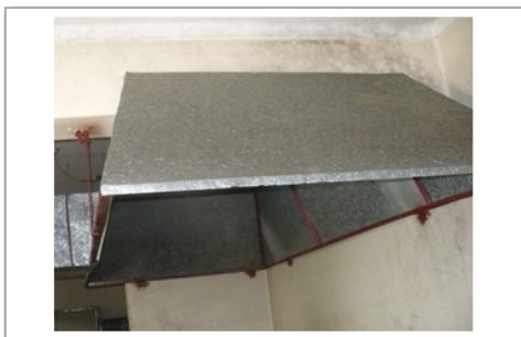
Renovation of NTS kitchen
