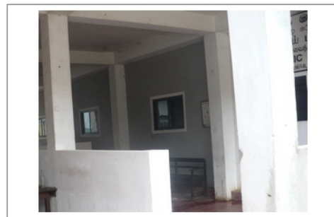
Construction of waiting area for Diabetic Patients
