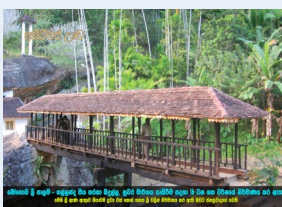
Bogoda Timber Bridge
