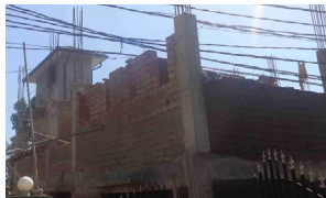
Construction of Radiology/ MRI building
