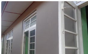
Operating theatre Repair
